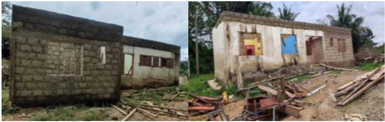
Renovated of Teachers Quarters at Dwirigum
